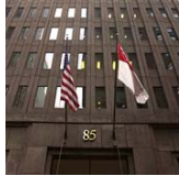
Goldman Sachs building at 85 Broad Street
